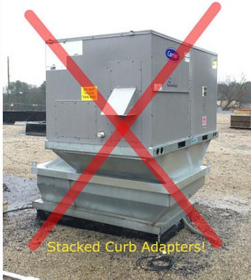
**Do not install a new curb adapter on top of an existing curb adapter. It can end up being unstable, extremely restrictive to airflow (which will result in all sorts of performance and service issues), will elevate the service compartment too high for normal access, and it will look like a HACK JOB.**
